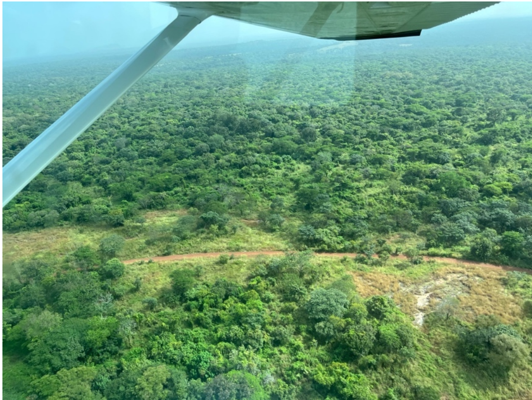
Figure 12: Observation of the road Tore-Rasolo.
